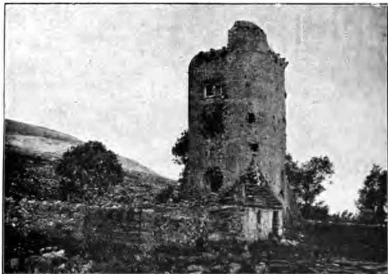
NEWTOWN CASTLE, BALLYVAUGHAN. (From the South.)
